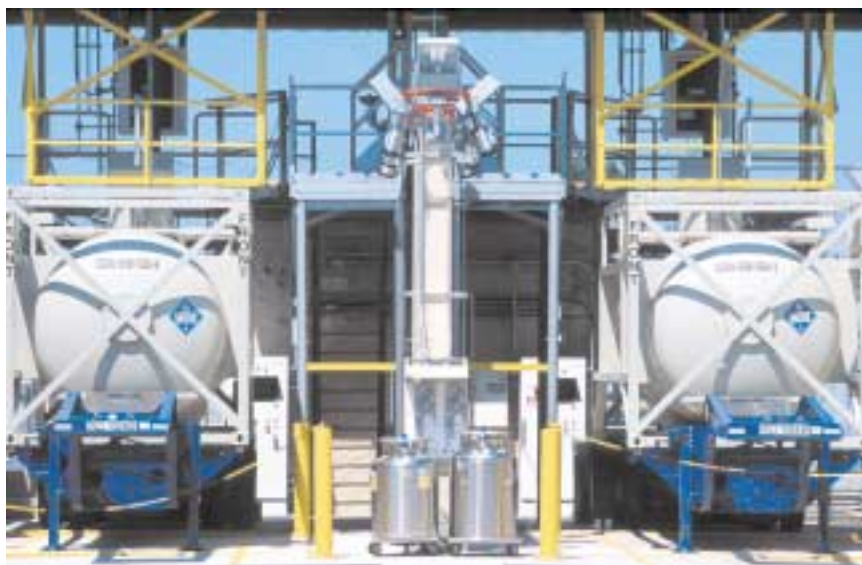
Figure 1. Scaling of specialty gas requirements associated with 300mm wafer processing may, in some cases, require use of bulk specialty gas systems (BSGS); a typical BSGS is shown.
