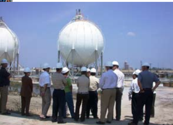
Staff from 16 electronics customers recently visited the Air Products' liquid hydrogen facility in New Orleans (NOLA) to see how the plant has quickly re-built from Hurricane Katrina.
