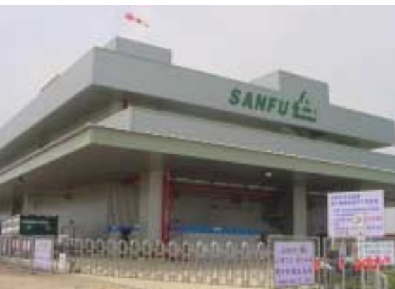
Air Products' Nanke ESG facility in southern Taiwan near Tainan serves the South Science Park and the rest of Taiwan and China.
