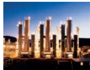
Located in western Wyoming, this nitrogen rejection unit processed up to 300 MMSCFD of EOR field gas for N 2 rejection and sales gas upgrading.
