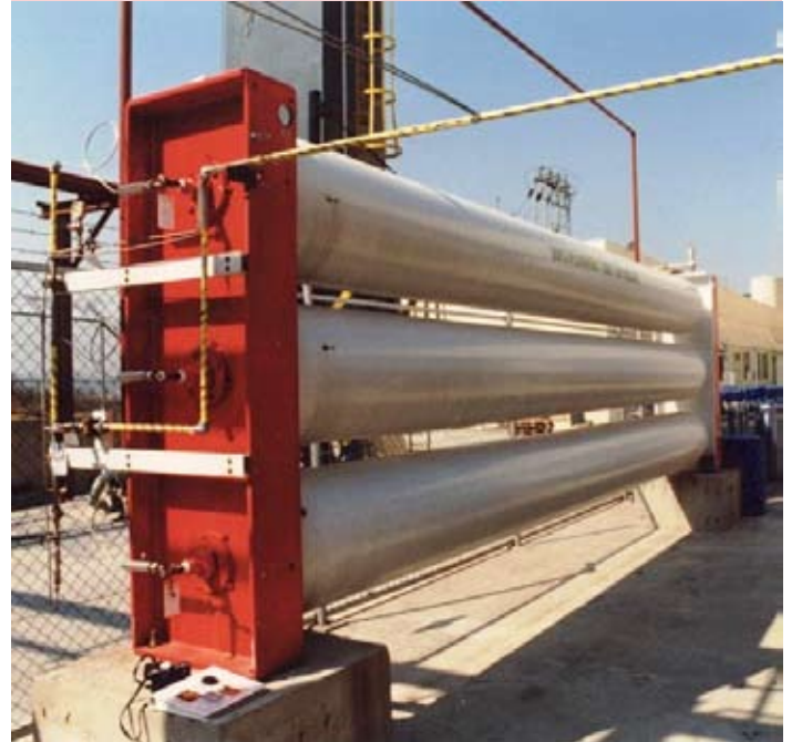
Typical Ground Tube Installation
