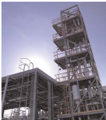
Air Products' new Ulsan, Korea UHP ammonia plant will serve customers in Asia and elsewhere.
