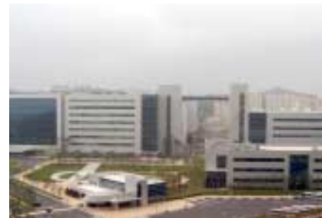
Air Products is a key supplier to Samsung Electronics' new Gen. 7 fab at Tangjung, Korea. It is the world's most advanced thin-film transistor/liquid crystal display (TFT-LCD) facility.
