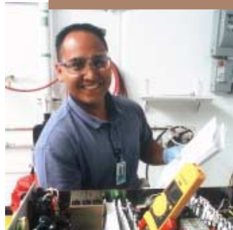
Technician Flo Bartoleme reviews test data while repairing a chiller at our Gilbert, Arizona facility.
