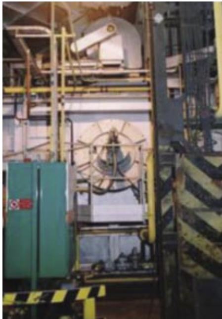
Figure 5: APMELT-RILEE™ technology and equipment, showing the high-temperature fan and burner/swirl chamber arrangement
