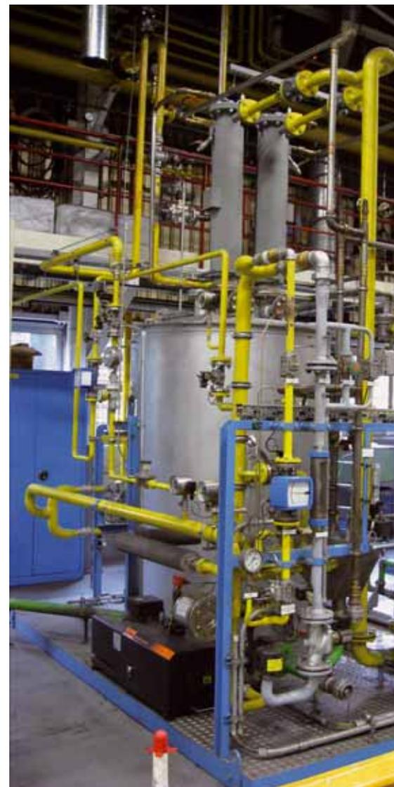
**Fig. 3:** Modified endogas generator
