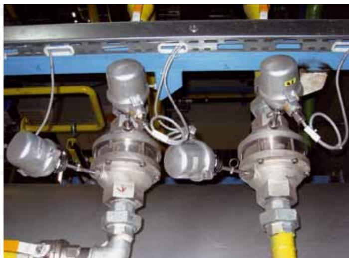
**Fig. 2:** Bidirectional, type-tested flame arresters
