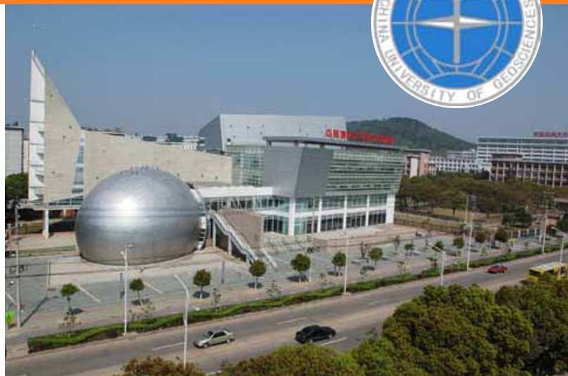
The Solar Energy Laboratory at the China University of Geosciences Wuhan.
