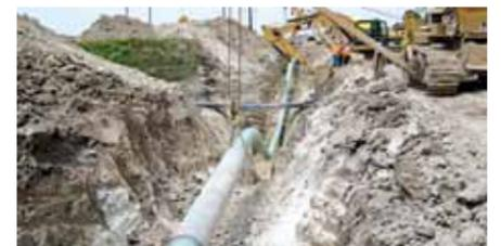
**FIG 3.** Laying Pipe for the Gulf Coast's new hydrogen pipeline.
