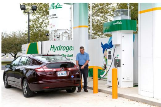
Air Products' SmartFuel® hydrogen fueling stations provide hydrogen fueling at 35 Mpa (5,000 psi) and 70 Mpa (10,000 psi) in compliance with JPEC (Japan Petroleum Energy Center) S0003. Use of the company's fueling technology is increasing and is already used in approximately 1,500,000 hydrogen fills per year. Air Products has been involved in over 200 hydrogen fueling projects in the United States and 20 countries worldwide.
