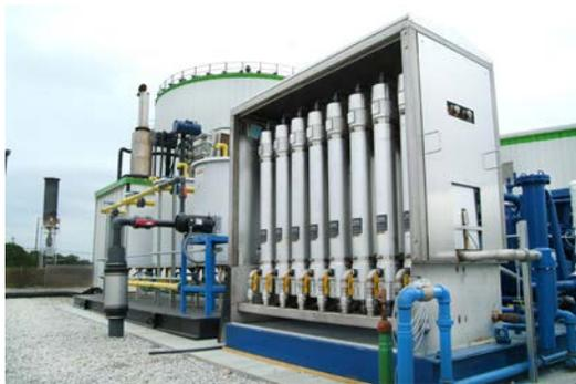
Air Products' PRISM® PB membrane separators have been used extensively for biogas and process gas upgrading facilities worldwide. The PB Membrane separators are PED certified to meet the Class-III requirements for safe flammable gas processing. This eliminates the need for secondary pressure vessels, making them a flexible alternative where space and access are limited.
