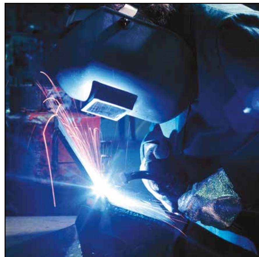
Cutting and welding
