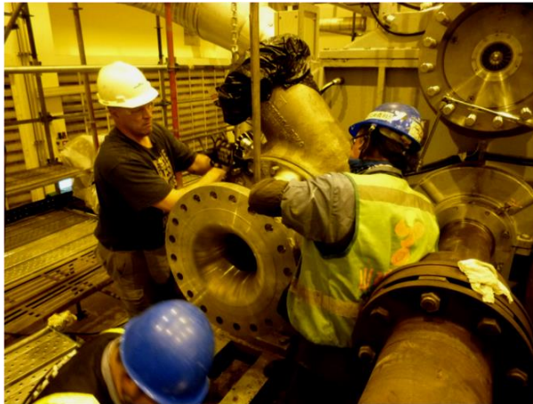
Centrifugal Compressor Inspection - Taiwan
