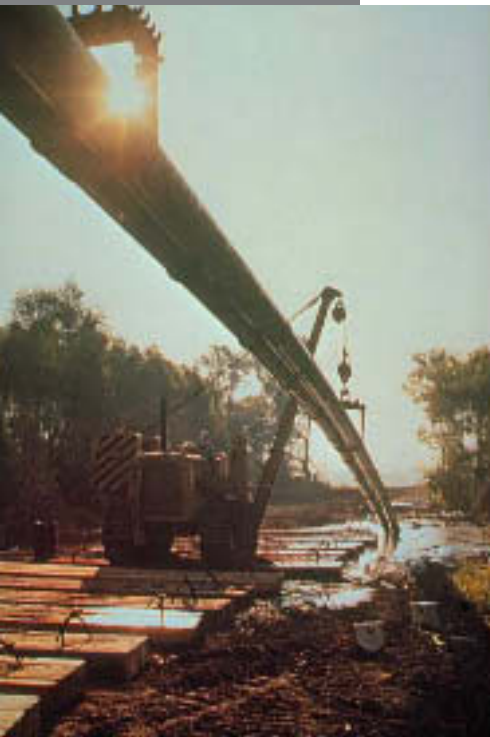
Directional drilling for the 1-mile (1.8 km) Mississippi River crossing pipeline.
