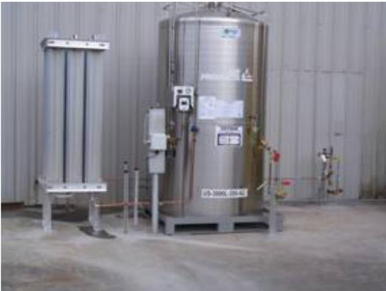
Your shop after CryoEase microbulk solutions . . . clean, efficient and simple.
