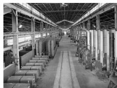
In 1944, Air Products moves to Chattanooga, Tennessee and produces 240 oxygen generators for the armed forces and for “lend-lease” to foreign allies. **Pictured:** Mobile and stationary oxygen generators under construction in Chattanooga.
