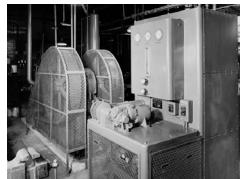
Air Products leases its first oxygen gas generator to a small Detroit steel company in 1941. **Pictured:** Grede foundries plant, Milwaukee, Wisconsin. An R-750 generator, typical of generators sold and leased in the 1940s and 1950s.
