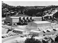
In support of America's emerging missile and space program, Air Products builds plants capable of producing tonnage quantities of liquid oxygen and nitrogen. **Pictured:** The Santa Susana Plant, featuring four 75-ton-per-day oxygen generators. It was, as Leonard Pool told his employees, "the largest single contract in [the company's] history."
