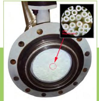
A PRISM Membrane separator contains thousands of fibers, which are bundled and encased at one end in epoxy resin. The bundle of fibers is inserted in a coded pressure vessel to provide correct flow distribution and pressure segregation.
