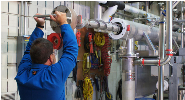
Vacuum-insulated conveyor
